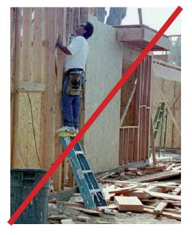
Don't use metal, wet wooden or fiberglass ladders to do electrical work. Wet ladders can make the ladder conductive to electrical current and creates slip and fall hazards.
